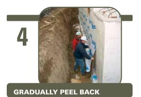
the remaining silicone release film, making sure the membrane is completely adhered.
